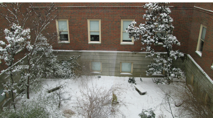
BEFORE | Pearson Hall's underused courtyard was transformed into a bright and airy internal atrium space (above).
